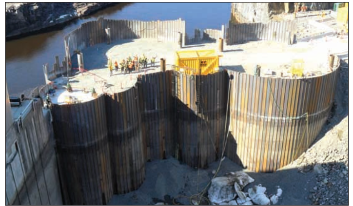
The cofferdam at Little Long GS was completed this April.
