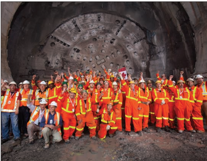
As Big Becky breaks through the last of its 10.2-km route under the City of Niagara Falls, employees of Strabag, the Tunnel contractor, celebrate the safe completion of the project’s excavation phase.
